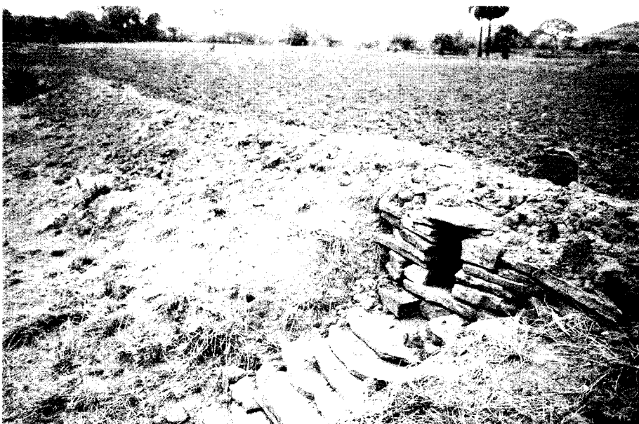
Traditional spillway with apron (drop structure) in Kenbarte - Kyaukpadaung
