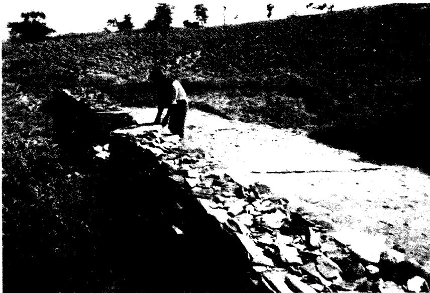
Stone checkdam full of sediments after rains
