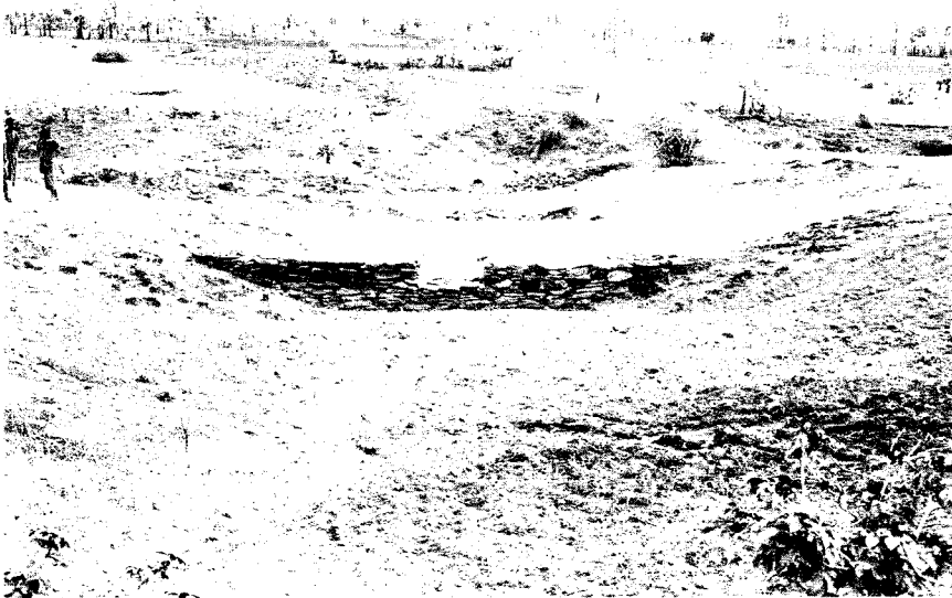
Stone checkdam across a small gully in Yaw Gyi Taw - Kyaukpadaung
