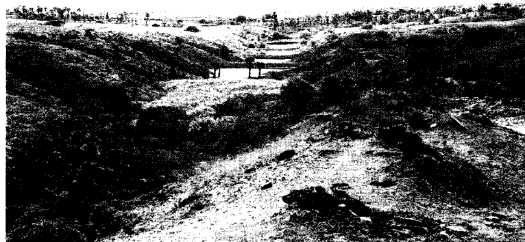
SS dams in series (the ones in the upper part full of sediments and already cropped the first season) in a deep and large gully in Yar Gyi Taw - Kyaukpadaung
