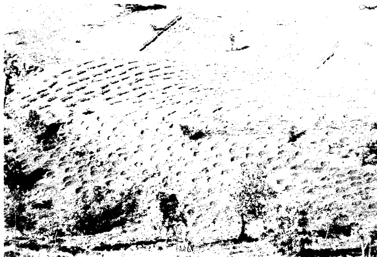
Hillside treated with microbasins on its steeper and upper portion, with trenches on medium slopes and soils bunds on gentle slopes (integrated rehabilitation)
