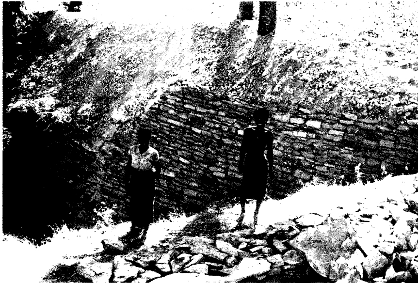
Traditional SS after renovation (right side of the stone wall), raising of the embankment and improvement of spillway in Thoine Kone - Kyaukpadaung.
