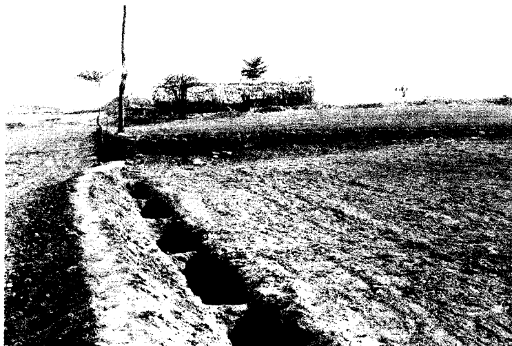
A strong boundary bund constructed in (Thee Kone - Kyaukpadaung)
