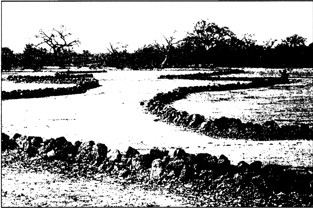
Stone lines set out on the contour (Burkina Faso)
