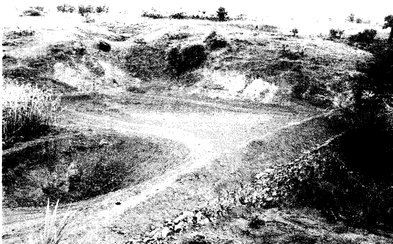
SS dam under construction (note the reshaping and creation of a new field where before was only a deep gully)
