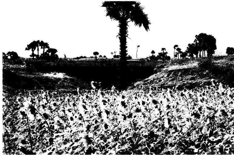
SS dam after construction (see also lateral protection of cultivated fields) in Thoine Kone - Kyaukpadaung
