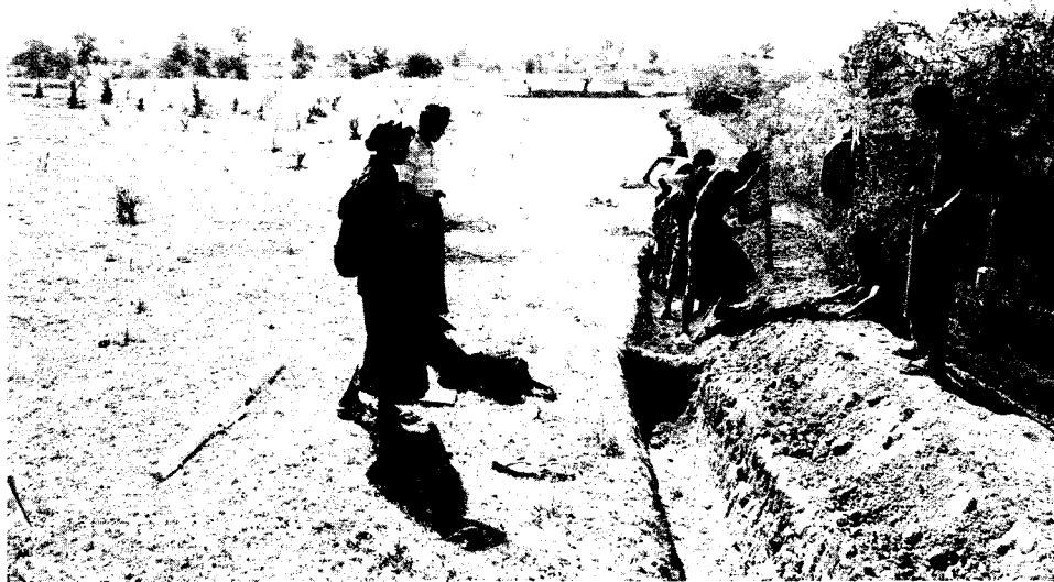
Bund under construction and compaction (Chaung-Ma-Kyaukpadaung)
