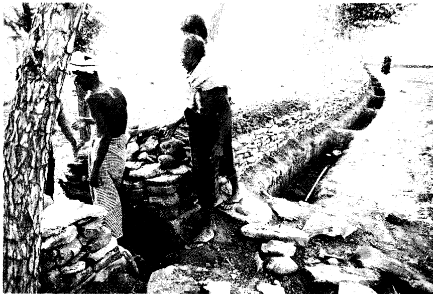
Double stone faced soil bunds with spillway under construction (Li Pin - Kyaukpadaung)
