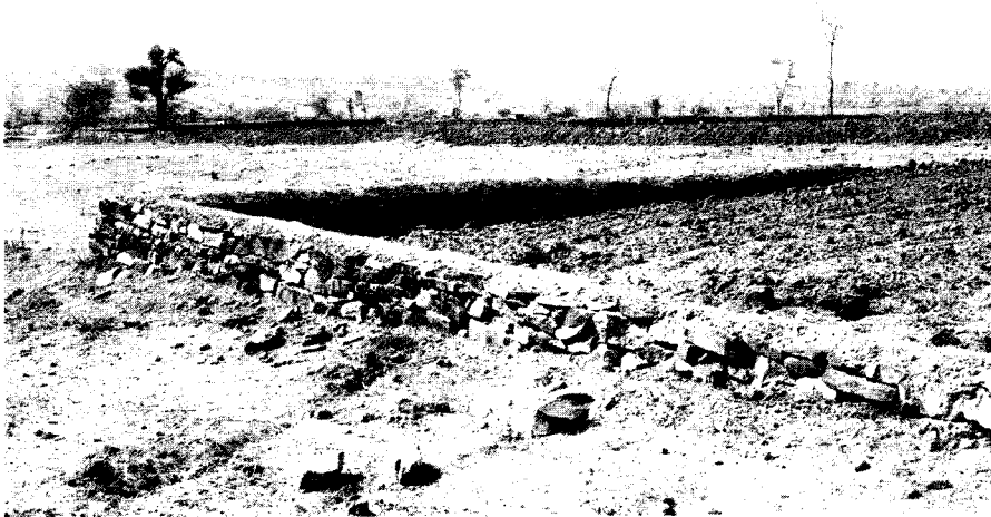
Example of "corner" or lateral bunds (Thee Kone - Kyaukpadaung)
