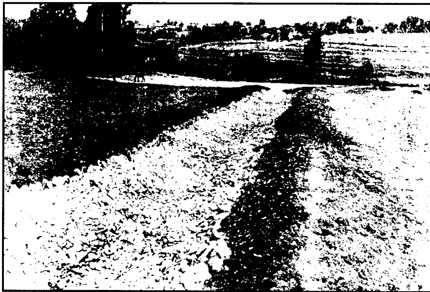
Example of a stone riprap waterway - (Ethiopia)
