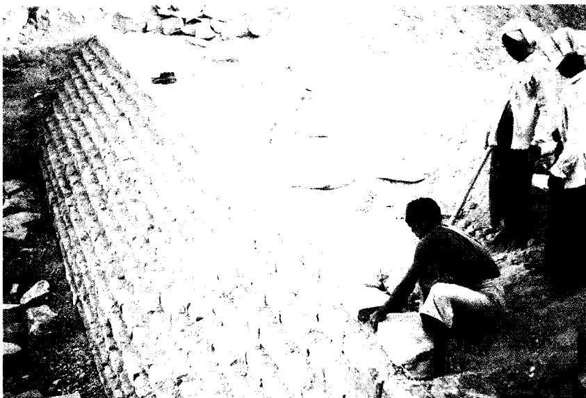
SS dam under construction (observe the accurate positioning of the stones)
