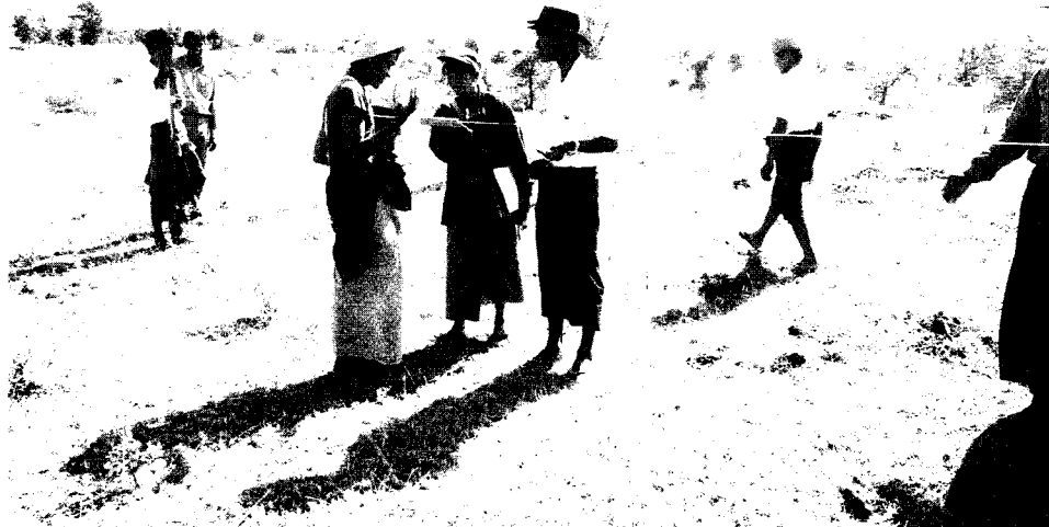
Layout of bunds using line level
