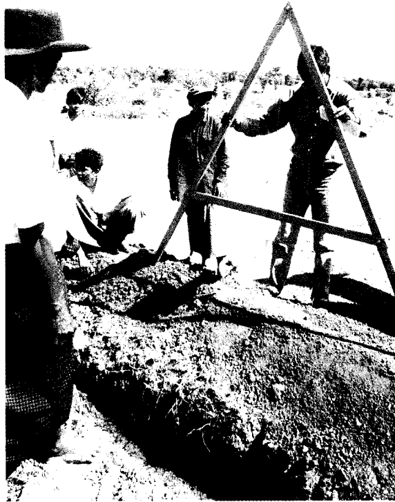
Checking the level of the top of the bund
